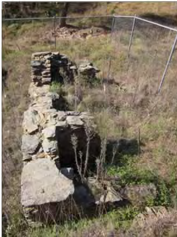
PLATE 5.5 May 2012 photograph of second stone structure, view to east
