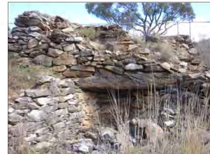
PLATE 5.2 May 2012 photograph of kiln structure, view to west
