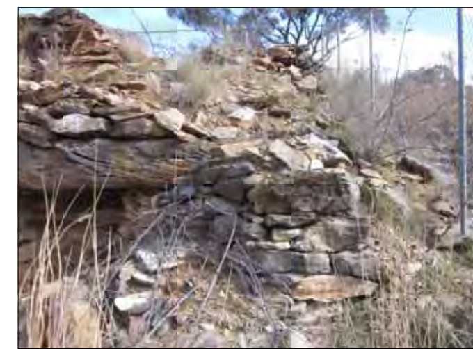
PLATE 5.3 May 2012 photograph of kiln structure, view to west
